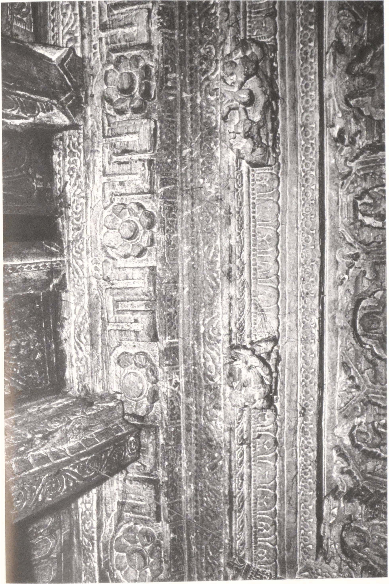
40 Upper part of the east façade, Ribba (photograph Christian Luczanits, WHAV LCH94 103,21)
